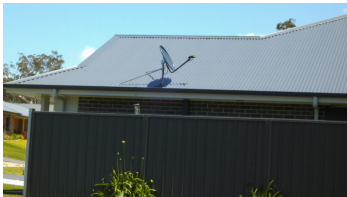
23. External TV antennas and dishes should be located at the back of the dwelling
