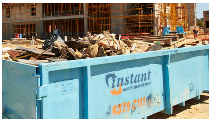
5. Skip bins must be utilised during construction
